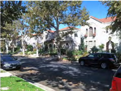
Walk-up rental four-plex buildings in a traditional neighborhood setting. These structures, in the Hancock Park neighborhood in Los Angeles, illustrate how small multi-family structures can present the quality and appearance of a single-family neighborhood. Streets like these are suggested later in this chapter as a buffer between single-family subdivisions on the west side of Gardner and the eastern edge of industrial development around the intermodal facility.
