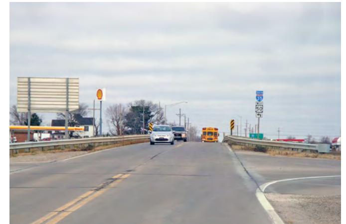
Gardner Road at the interchange with I-35
