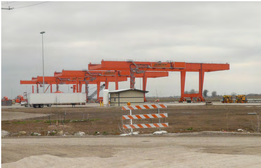
BNSF Intermodal Facility KC
