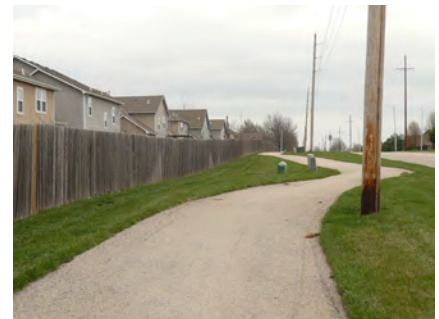
Center Street and 183rd Street sidepaths in Gardner.
