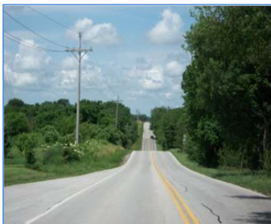
Improvements west of K-10 would address more long term needs. (Existing shown)
