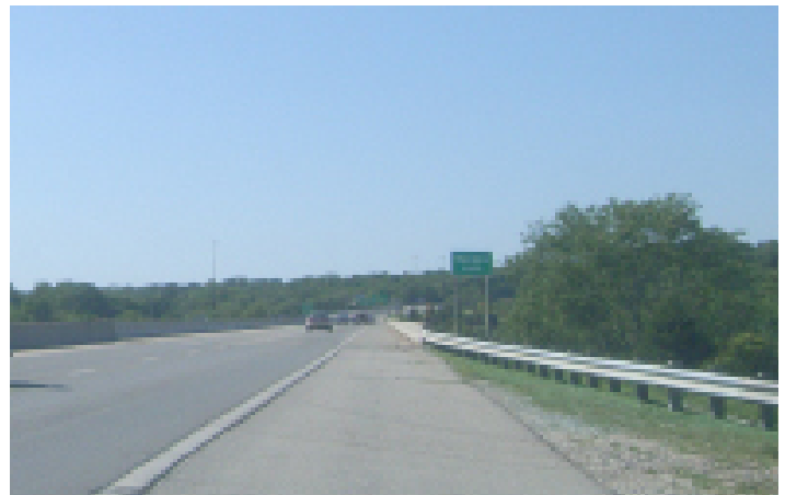
Existing Northbound K-7 Bridge over Kansas River
