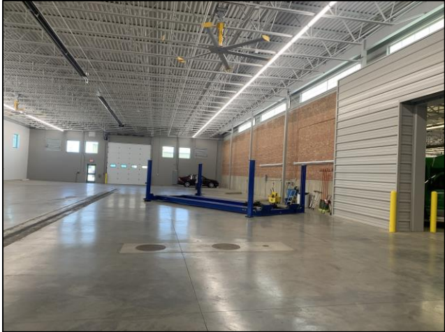
Figure 8: Newly Constructed Vehicle Storage and Repair Area (Photos: TranSystems)
