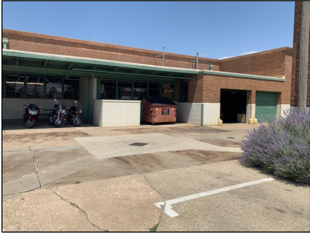
Figures 9 & 10: Concrete Wear Examples Surrounding Facility (Photos: TranSystems)
