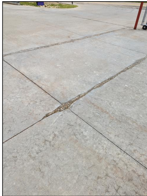
(Location: South of Main Entrance)
