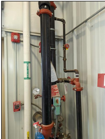
Figure 4 & 5: Sprinkler System Shutoff and Fire Extinguisher Example (Photos: TranSystems)
