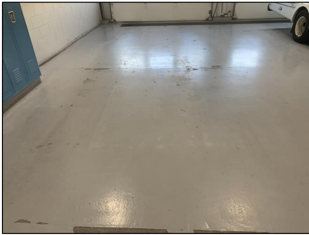
Figures 8 & 9: Concrete Wear Examples Surrounding Facility (Photos: TranSystems) (Location: West of Maintenance Facility)
