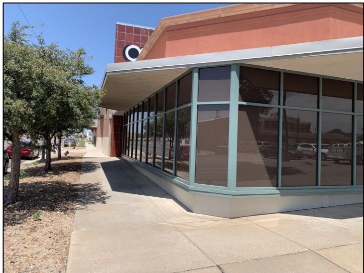
Figure 1: OCCK, Inc. Administration and Maintenance Facility (Photo: TranSystems)
