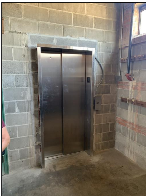
Figure 5: Elevator Example (Photo: TranSystems)
