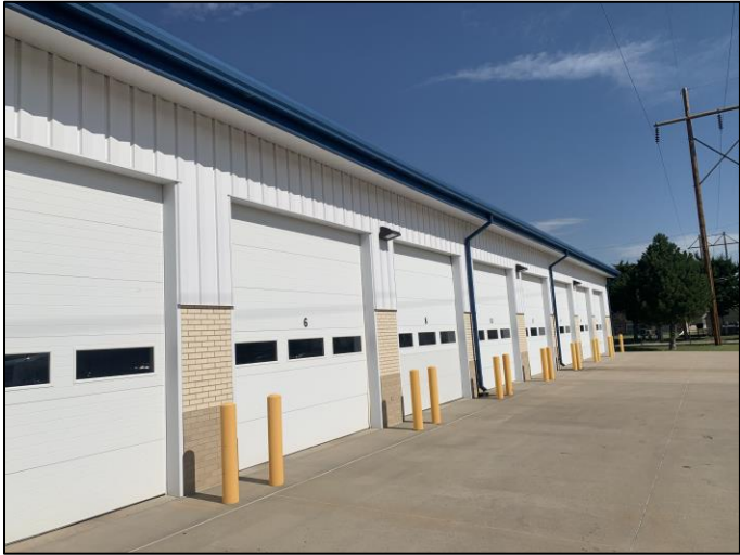
Figure 4: Exterior of Vehicle Storage Door Example (Photo: TranSystems)
