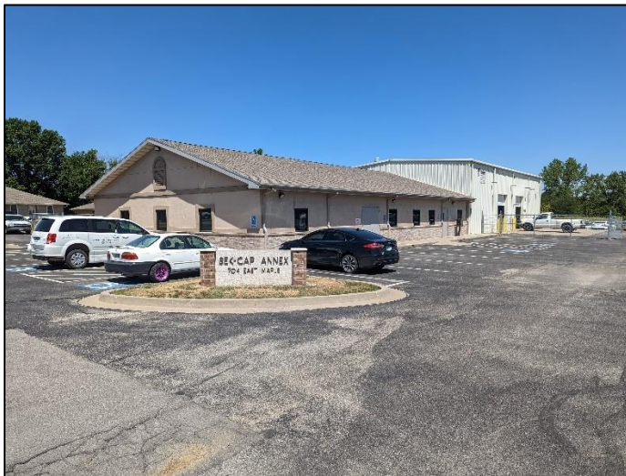
Figure 1: SEK-CAP Facility (Photo: TranSystems)
