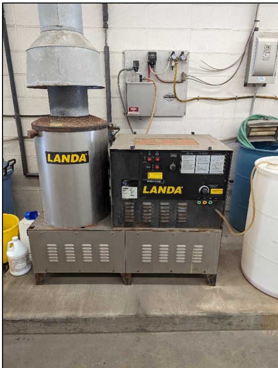
Figure 4 – 5: Wash Bay Water Pump, Heater and Water Pipe Corrosion Example (Photo: TranSystems)
