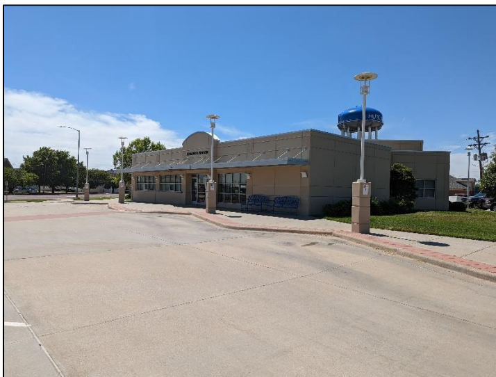
Figure 1: RCAT Facility (Photo: TranSystems)
