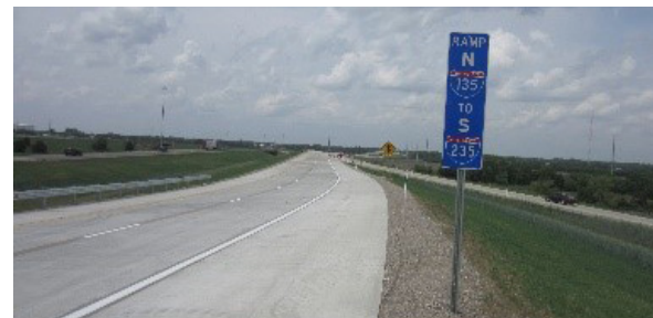
I-135 to I-235 Flyover Bridge Project Sedgwick County
