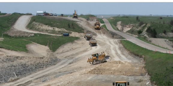
U.S. 281 Modernization Russell County
