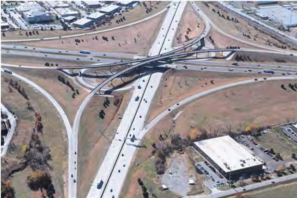
Johnson County Gateway Project – I-435 • I-35 • K-10
