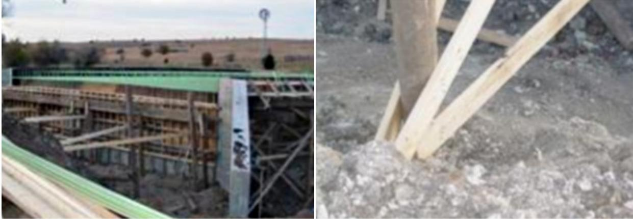
**Figure 11: Driven Posts and Strongbacks**
