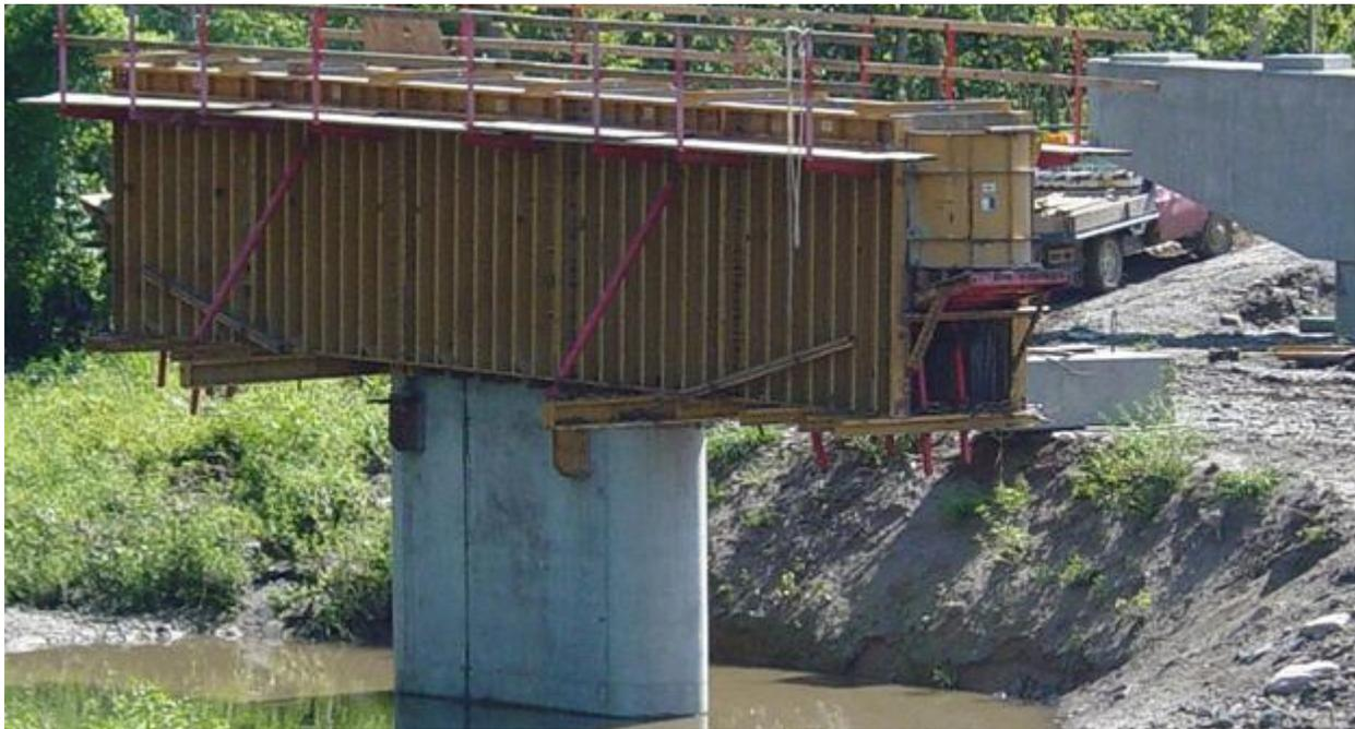
**Figure 16: Plate Girder Form System**
