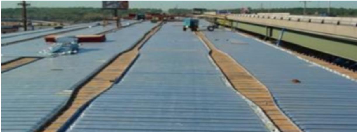
**Figure 14: Steel SIP Form Installation**
