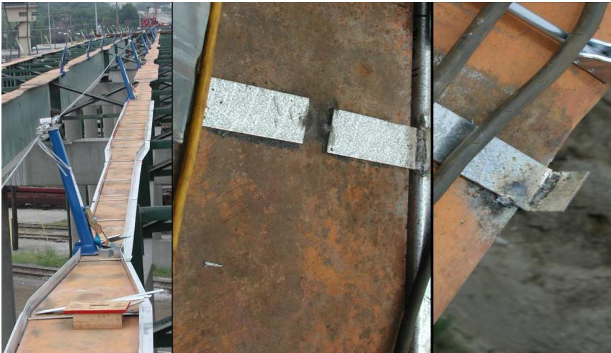
**Figure 15: SIP "ladders" Welded In Place**
