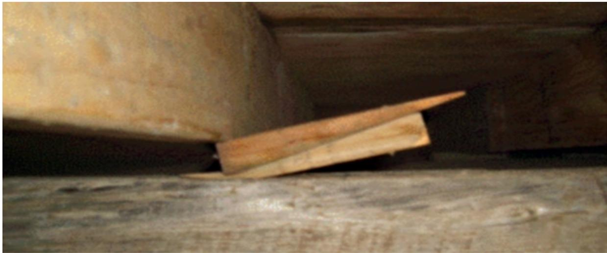
**Figure 20: Incorrect Shim Placement**
