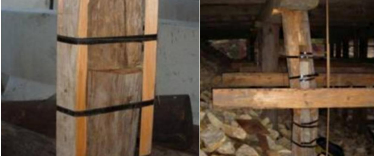
**Figure 19: Potentially Dangerous Column Splice Details**
