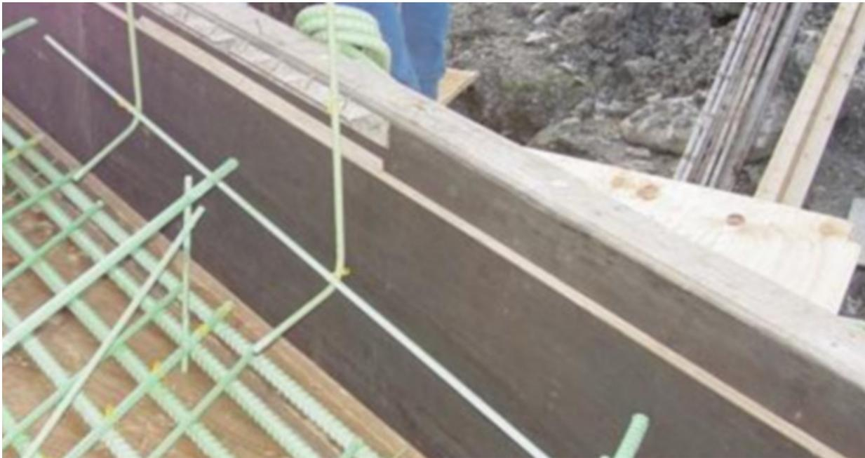
**Figure 20:  $\frac{3}{4}$ " Triangular Chamfer Strip**
