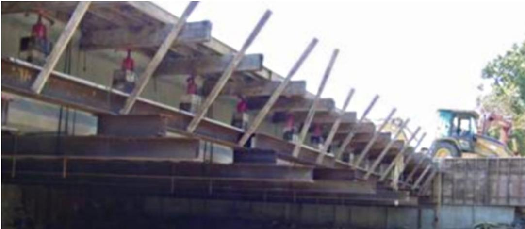
**Figure 8: Needle Beam Overhang Falsework**
