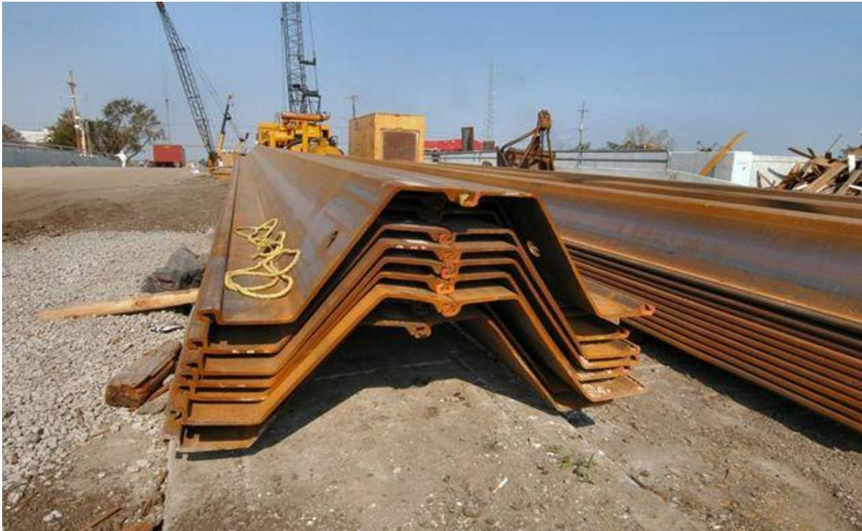
**Figure 4: Pre-coupled Z-shape Sheet Pile**
