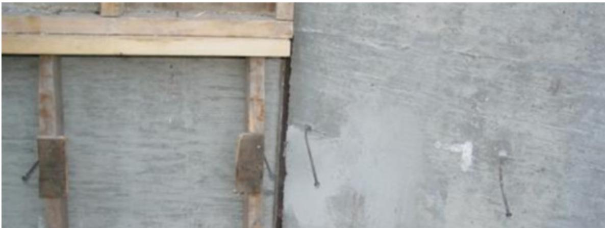
**Figure 10: Remaining Break Off Ties**
