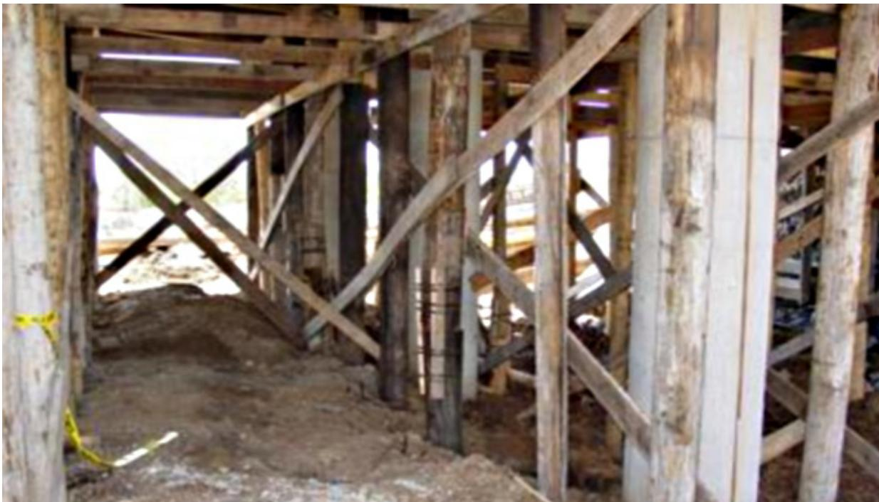
**Figure 18: Falsework Column Splice (Center)**
