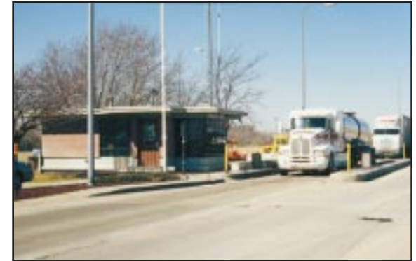
North Platte I-80 mainline WIM sensors
