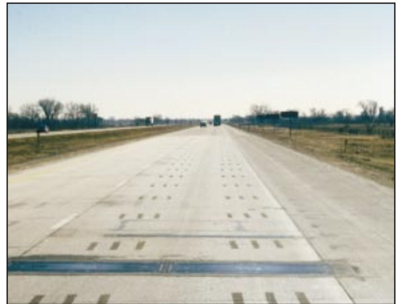
North Platte weigh-in-motion facility
