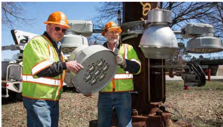
Figure 4: Technicians Lower the High-Mast Lights to the Ground Level for Re-Lamping Source: [11]
