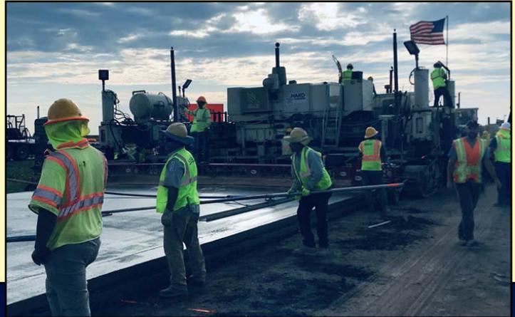
**Above:** crews are pouring the concrete overlay on the bridge at Ellis. **Top right and at right:** crews work place a new overlay on the bridge over I-70. Photos by Joshua Morales and Todd Anderson, District Three
