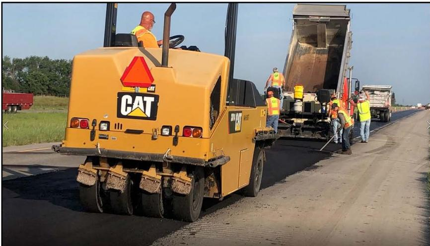
*In the photos at left and below, a team effort took place on Aug. 20 as crew members from the Council Grove Subarea assisted the McPherson Subarea place a cold mix overlay on the driving lane of a four-mile stretch of I-135 in McPherson County just south of Moundridge. Kort St. Clair, Highway Maintenance Supervisor in McPherson, said he hopes the overlay will smooth out the patches on the road and help to extend pavement life. Photos by Ashley Tammen, District Two*
