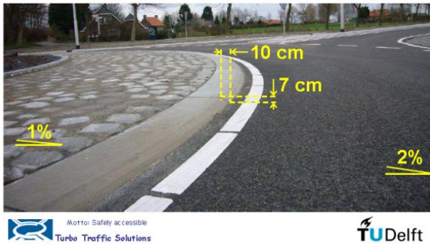
FIGURE 5.17 Cobblestone Truck Apron in Netherlands Showing Curb Height and Slopes
