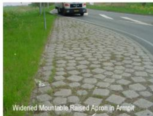
FIGURE 5.18 Cobblestone External Truck Apron in the Netherlands
