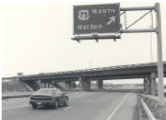
The US-75/US-24 interchange will be reconstructed as part of the US-75 work from the Westgate bridges to Soldier Creek.
