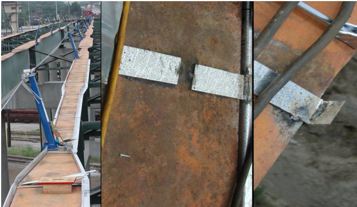
Figure 15: SIP "ladders" Welded In Place
