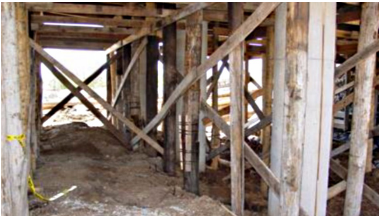
Figure 18: Falsework Column Splice (Center)
