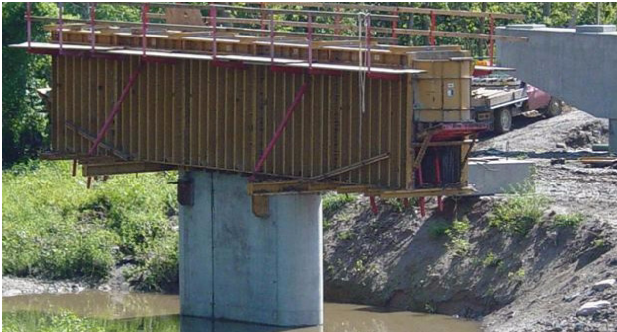
Figure 16: Plate Girder Form System
