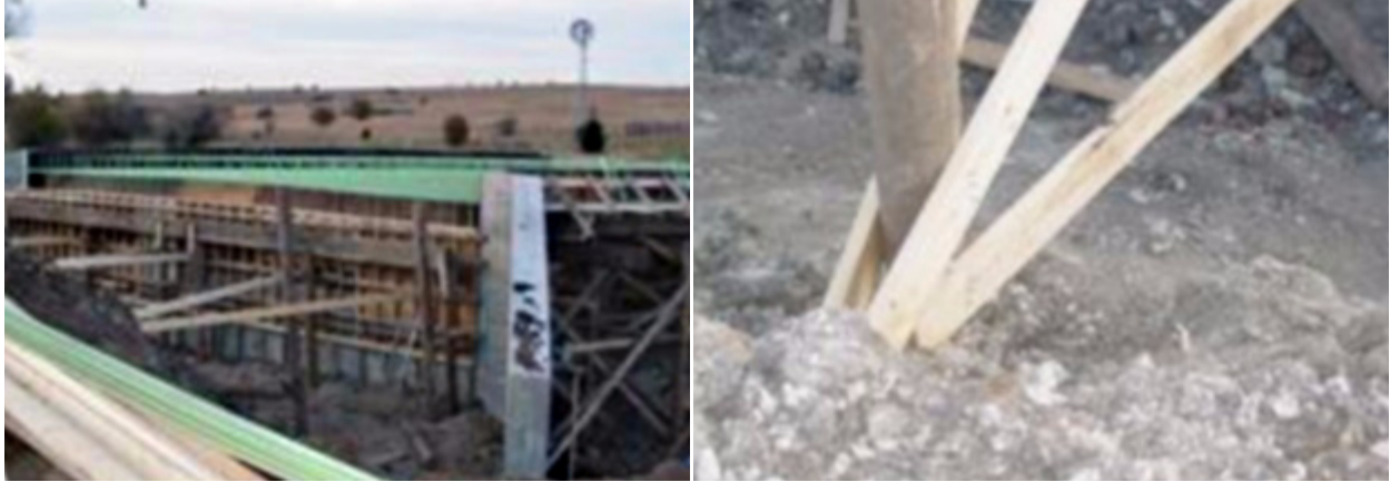
Figure 11: Driven Posts and Strongbacks
