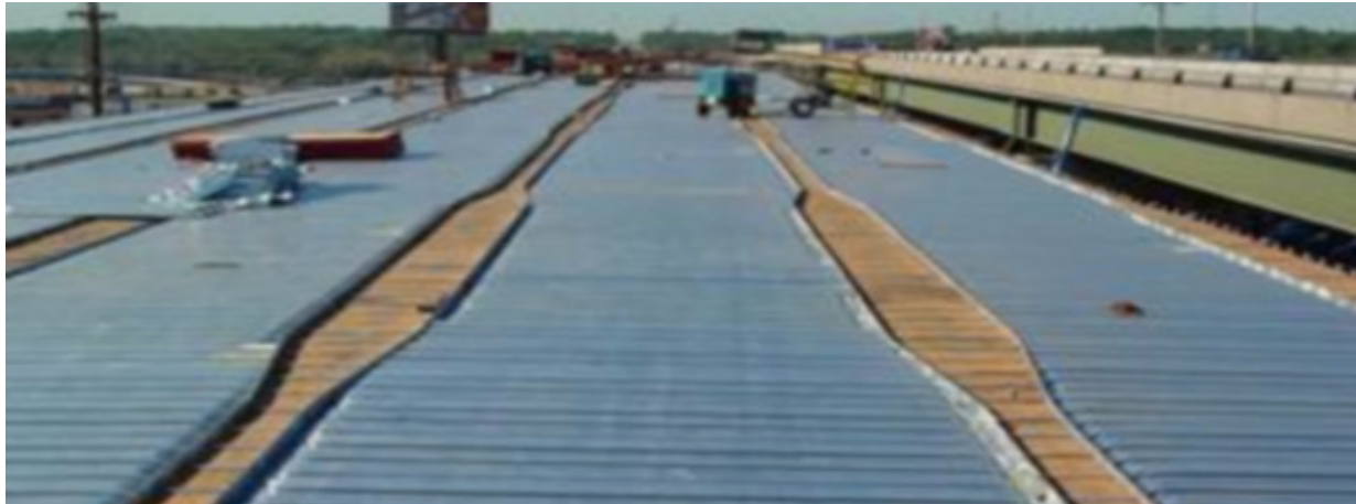
Figure 14: Steel SIP Form Installation
