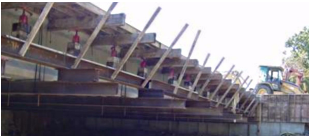
Figure 8: Needle Beam Overhang Falsework
