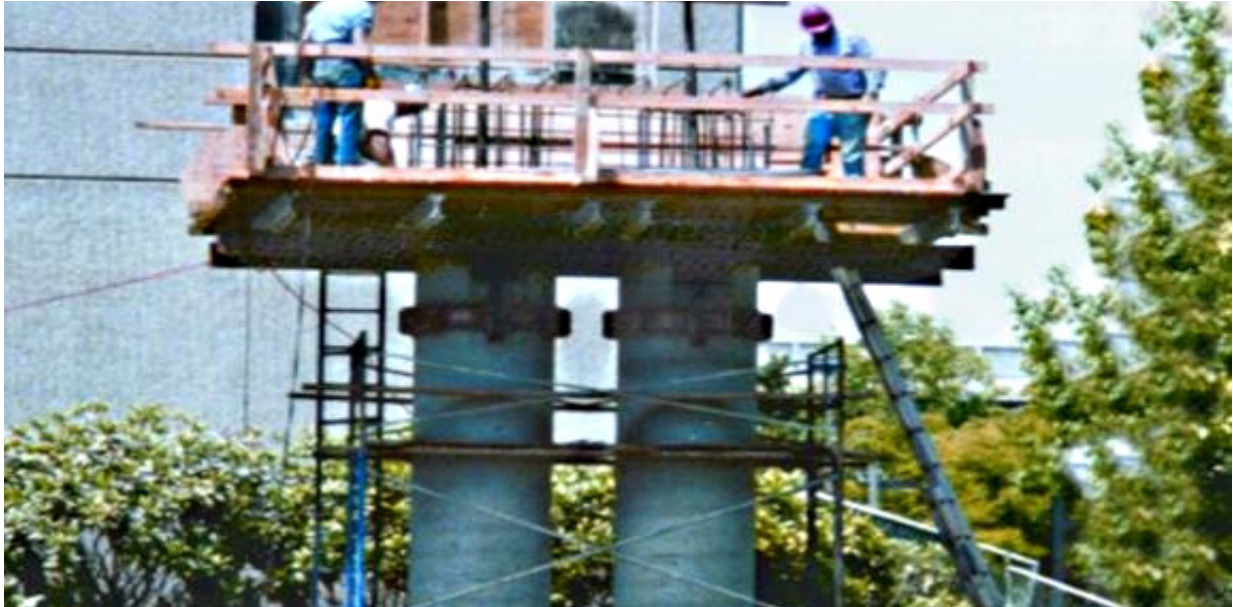
Figure 17: Friction Collars Attached to Columns
