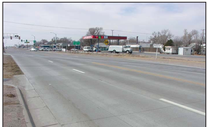
This project on U.S. 160 in Ulysses earned a partnering award from the Kansas Contractors Association and KDOT. Photo by Chuck Oldaker
