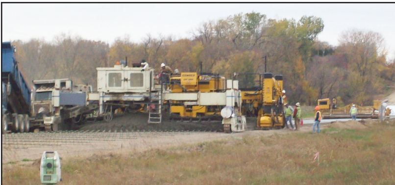
Pavement work is progressing on U.S. 24.
