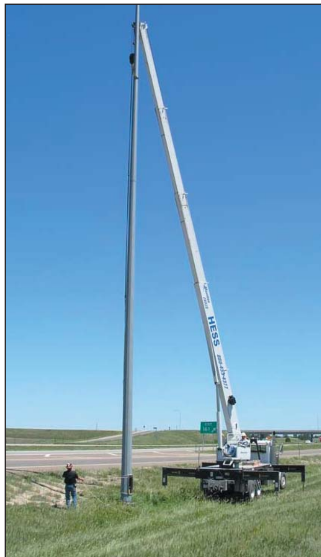
Above, a light pole is removed on I-70 near Exit 161 - the same day an 18-inch crack is discovered near the base of the structure by KDOT Equipment Operator Kent Huss. Below, only about two-thirds of the 18-inch crack in the light pole can be seen in this photo. Photos by Kevin Zimmer
