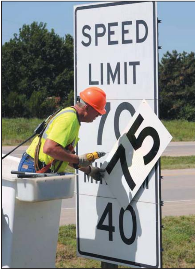
Equipment Operator Specialist Jeff LaCrone places an aluminum overlay on a 70-mph sign on I-70 near Topeka. The new 75-mph speed limit went into effect on 807 miles of roadway in Kansas on July 1. Photo by Kurt Weaverling
