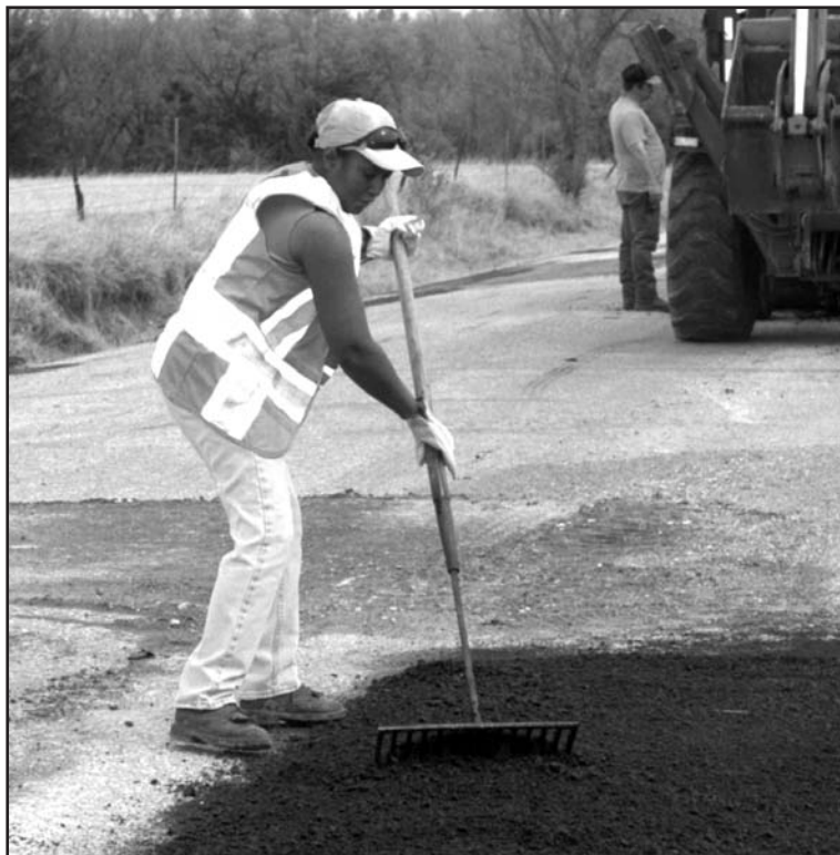
KDOT employee Irene Daniels smooths out asphalt during a patching project.
