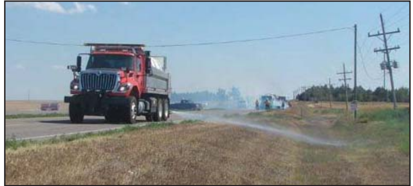
To reduce the risk of fire, a KDOT crew sprays water ahead of work taking place on U.S. 283 in Ford County.
