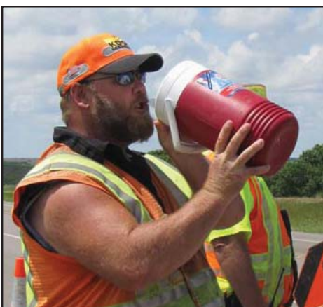
Equipment Operator Dave Kelley from Smith Center takes a quick break while working on spur route K-204.
