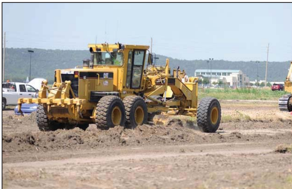
Grading work takes place along part of the K-18 project in Riley County.
