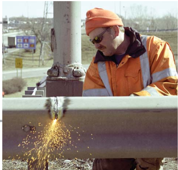
Jim Koerner, Equipment Operator in Wichita, uses a cutting torch to remove and replace the guardrail.
