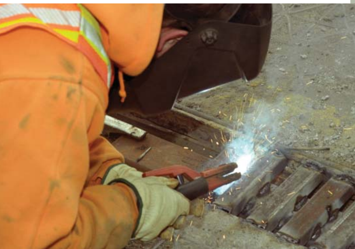
Welding work takes place on the existing U.S. 59 Amelia Earhart Bridge at Atchison.
