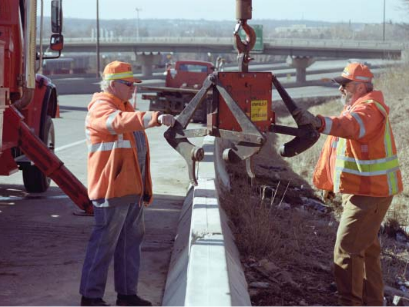
Bob Malay (left), Equipment Operator Senior, and Doug Essenpries, Equipment Operator, both from the Speaker Road Subarea, repair barrier along I-670 in Kansas City.
