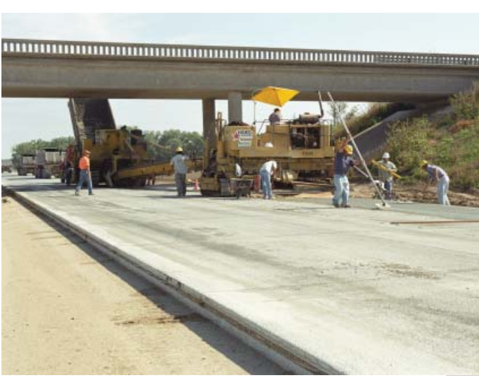
Cement is poured on the new I-70 lanes east of Salina.
