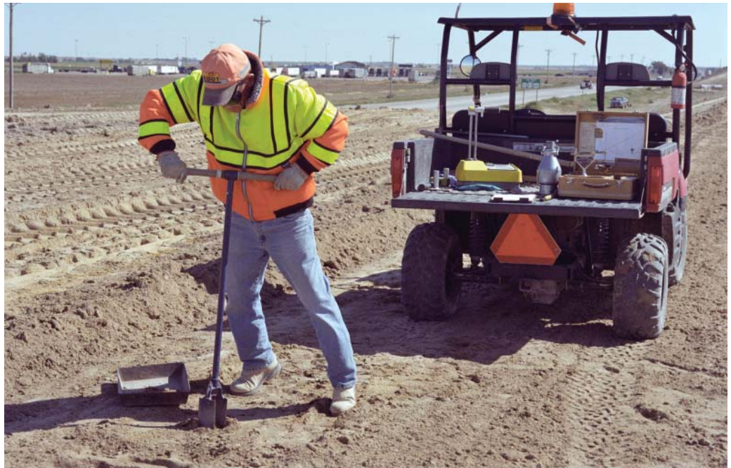
Engineering Technician Larry Kells takes a sample of the U.S. 50/U.S. 400 road base near Garden City to help assure the future road will have a good foundation.
