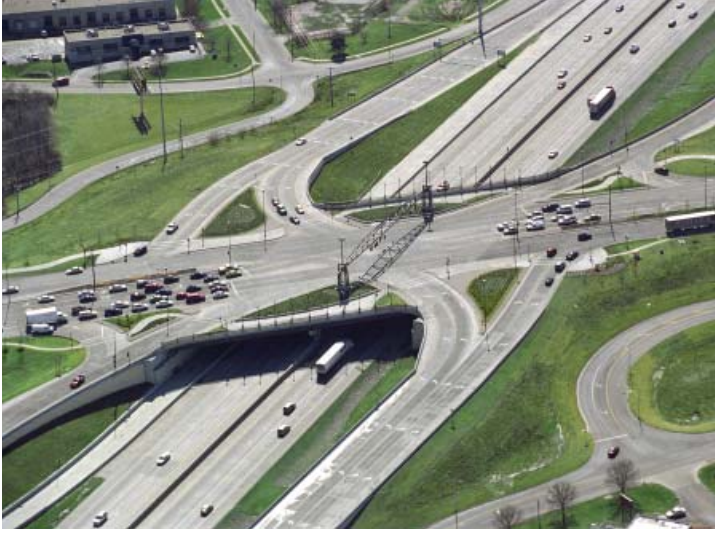
The Single Point Urban Interchange (SPUI) at the I-35/87th interchange in Lenexa greatly reduces congestion.
