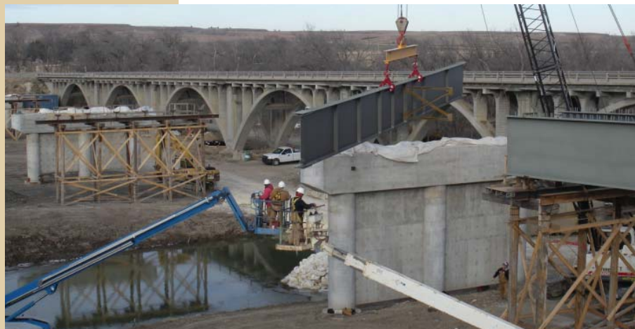
The new U.S. 183 Saline River Bridge will replace the narrow structure in the background.
