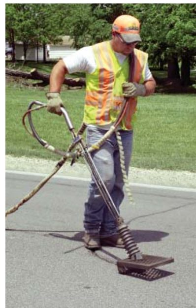
Equipment Operator Jason May from the Marion Area crew operates a heat lance while working on a crack sealing job on K-177 in Chase County.
