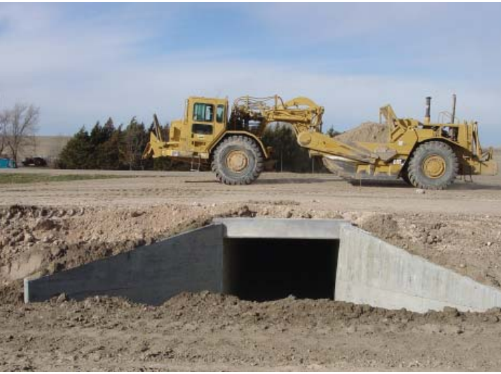
Grading takes place on a project to realign K-27 in Sherman County.
