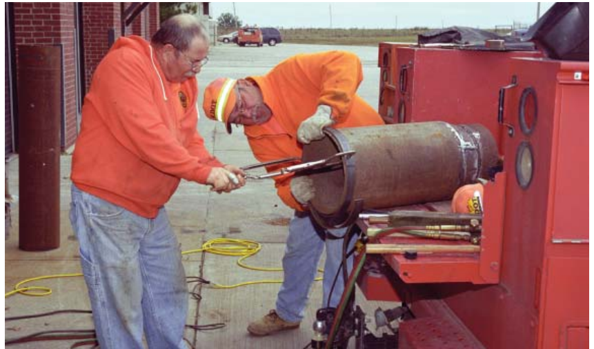
Winfield Area crew members Matt Groene, left, and Stan Schwantes construct a new fill spout for a salt dome.
