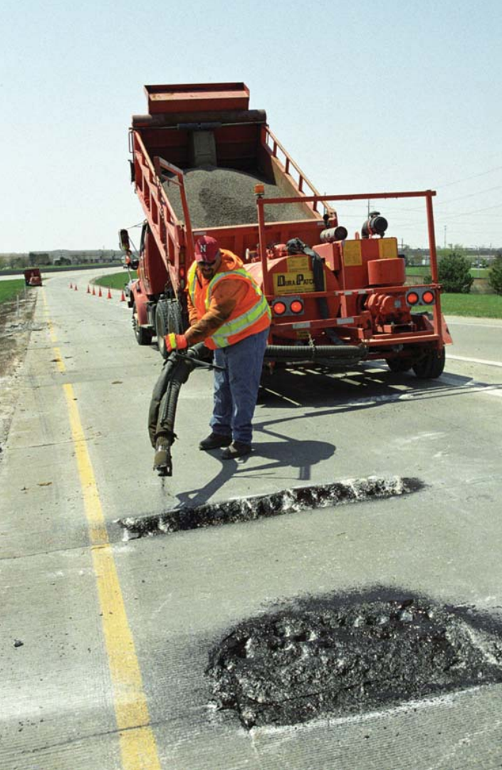
Equipment Operator Thomas Mallon Jr. of the Gardner Subarea repairs pavement failures on I-435 with a spray patcher.
