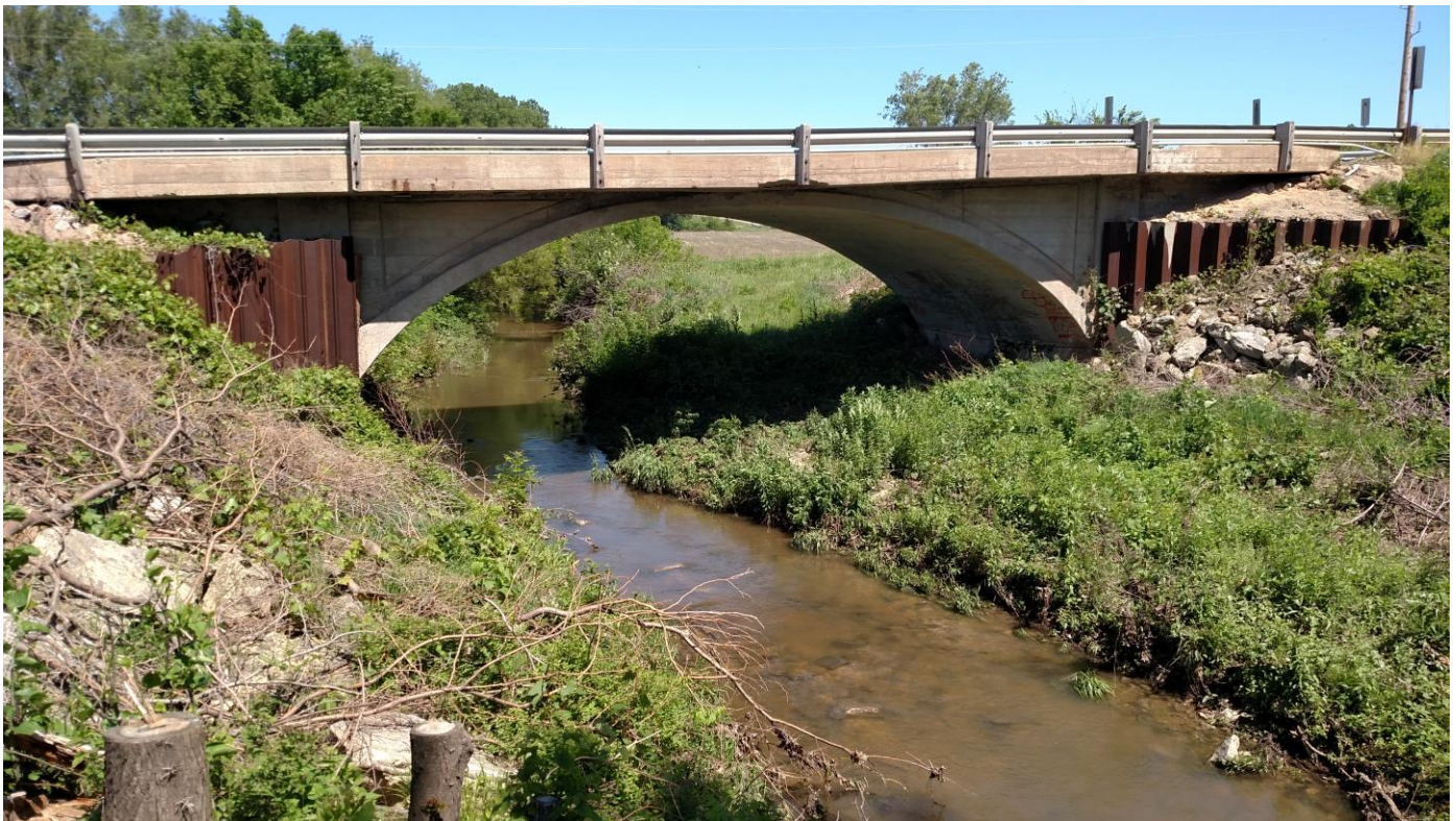
A current view of existing K-63 Bridge over Straight Creek.
