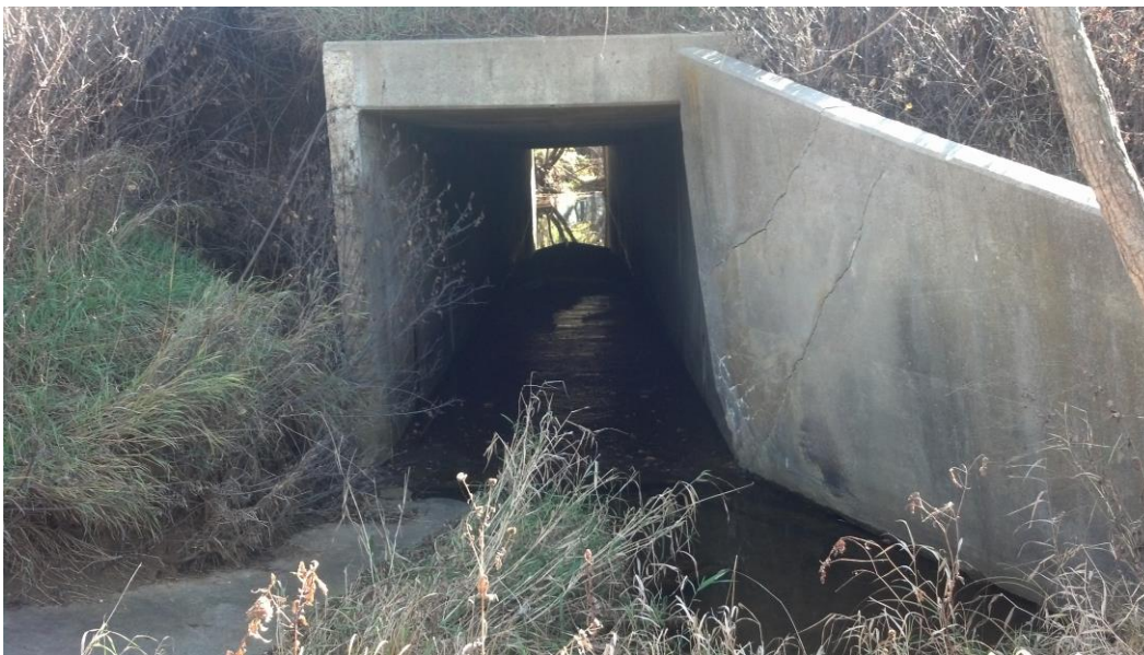
A current view of existing concrete box culvert under U.S. 36.
