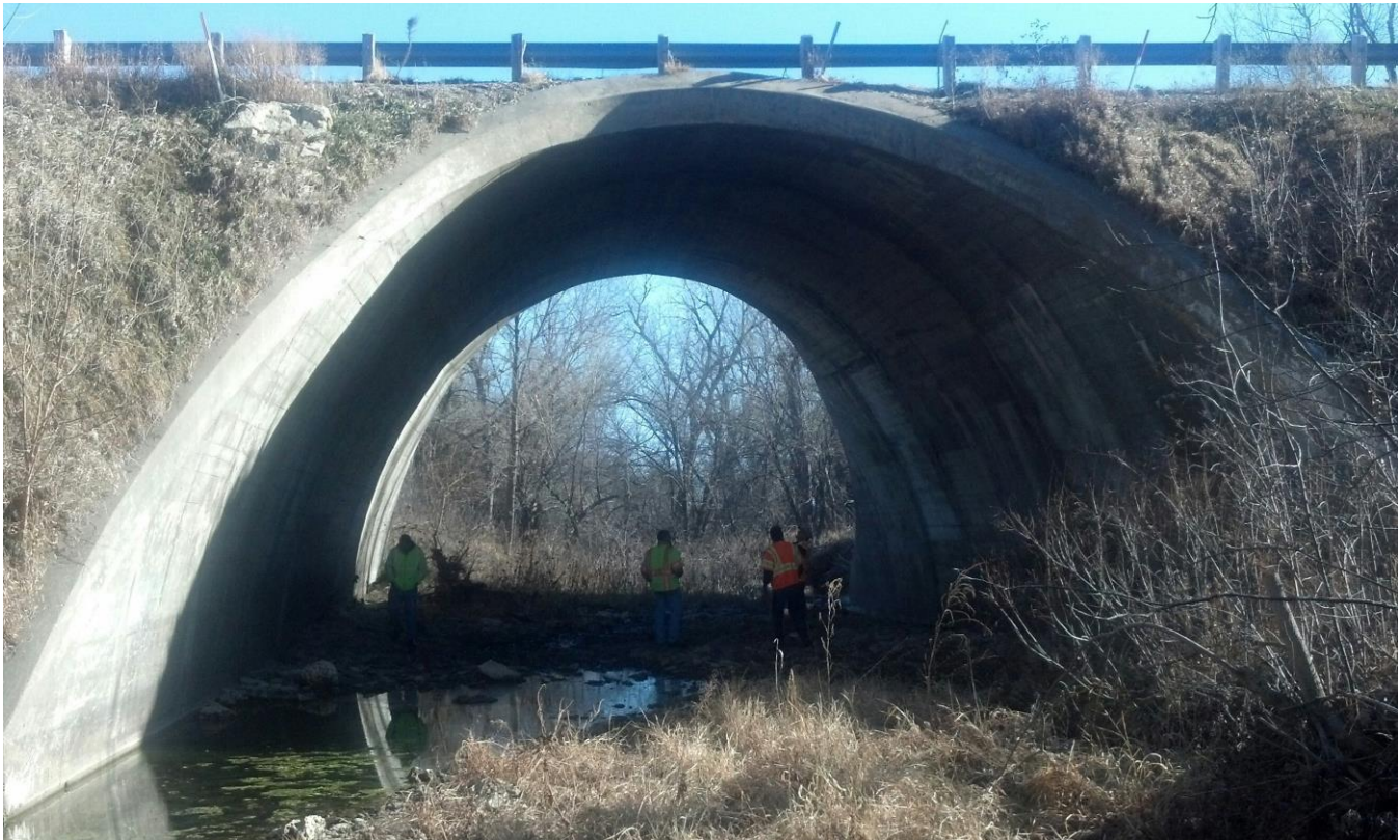
A current look at the existing U.S. 77 Swede Creek Bridge.
