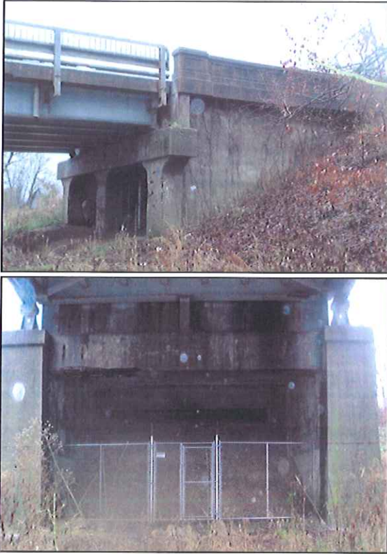
Photo 12 and 13: Bridge Design Mimicking "Cave-like" Atmosphere
