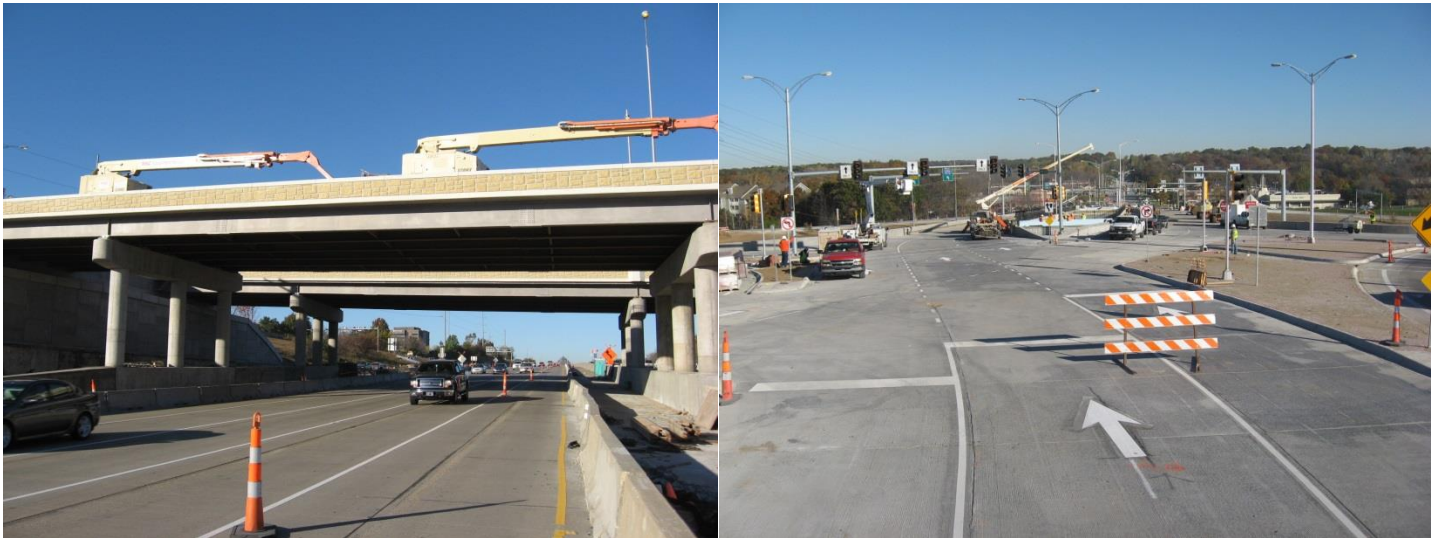
Today's view from I-435 of the new Roe Avenue bridges (left). A Roe Avenue view of the DDI movement across the new bridges over I-435 (right).
