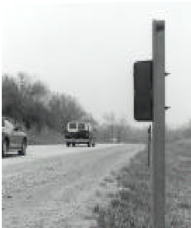
Warning reflectors on K-4 in Shawnee County have shown success in reducing deer-vehicle accidents.
