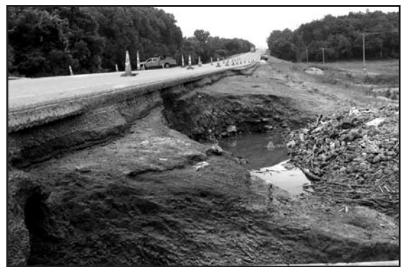
Above and middle right: US-59 north of Garnett was severely damaged by flood waters July 1. Emergency work took place and the roadway is repaired.
