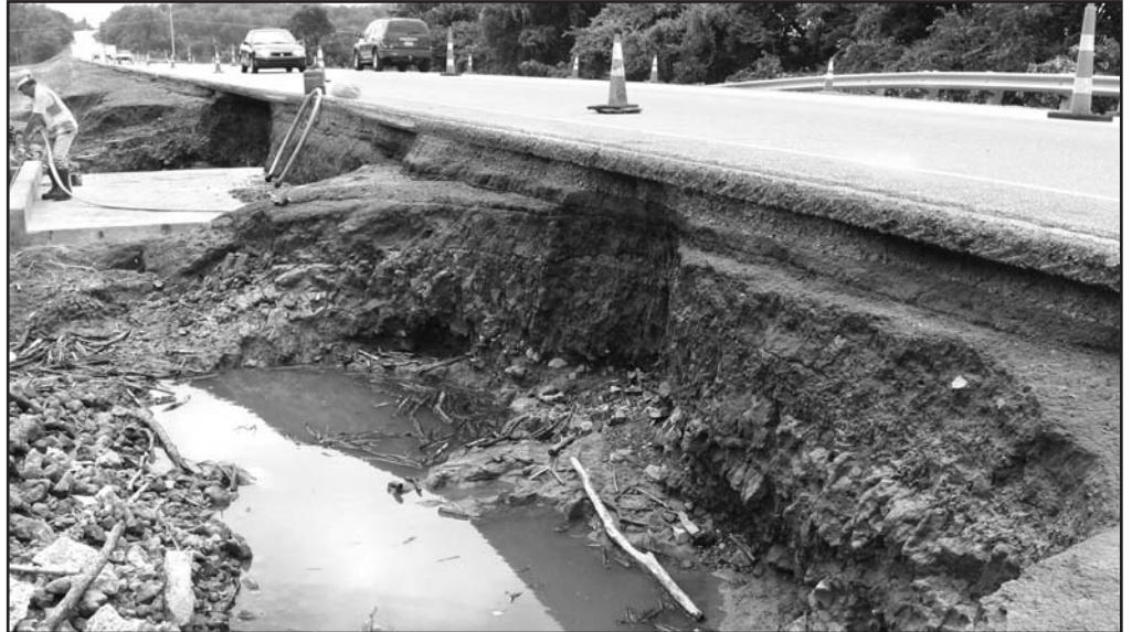
Above and middle right: US-59 north of Garnett was severely damaged by flood waters July 1. Emergency work took place and the roadway is repaired.
