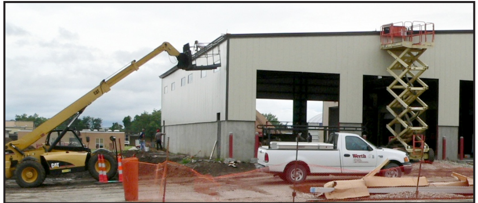
Work continues on the Ellsworth Subarea building. Photo by David Greiser
