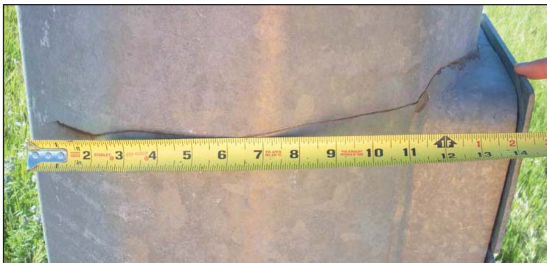
Above, a light pole is removed on I-70 near Exit 161 - the same day an 18-inch crack is discovered near the base of the structure by KDOT Equipment Operator Kent Huss. Below, only about two-thirds of the 18-inch crack in the light pole can be seen in this photo. Photos by Kevin Zimmer
