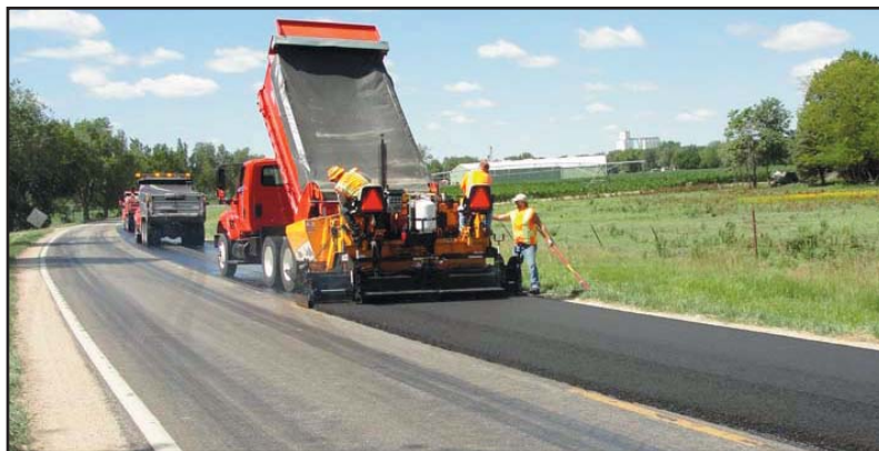
Asphalt overlay work takes place on K-89 in Harvey County.
