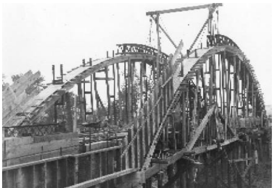
The Republican River Marsh Arch bridge was under construction near Fort Riley during this 1918 photograph. The bridge was the first highway project in Kansas to receive federal aid.
