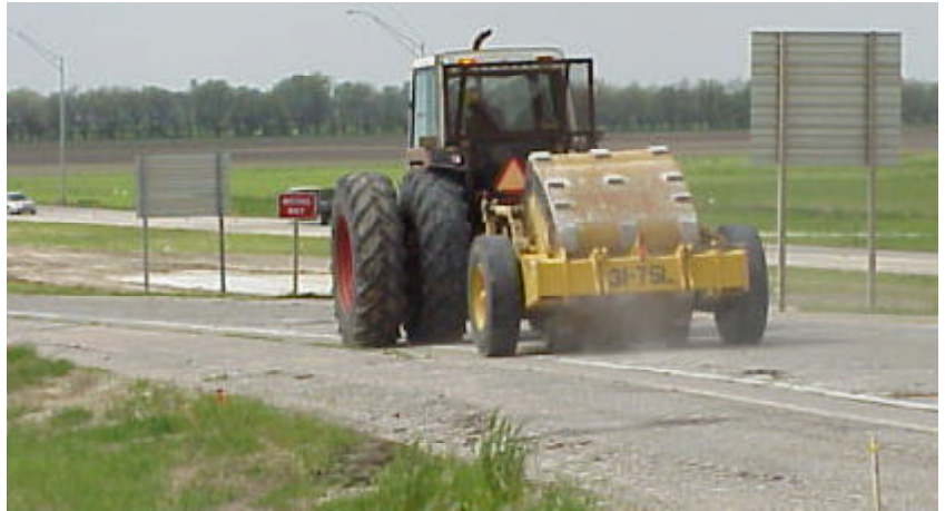
KDOT received a national award for this work on I-135.
