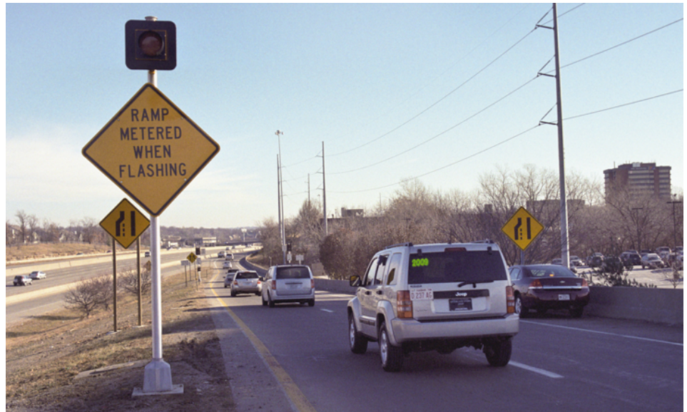
Ramp metering is being used at locations on I-435 in southern Johnson County to help motorists deal with traffic congestion. Photo by Kurt Weaverling
