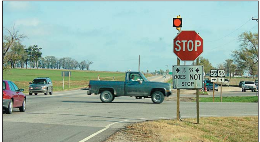
One of several safety features includes a flashing beacon on a stop sign alerting drivers on US-56 that US-59 traffic does not stop.
