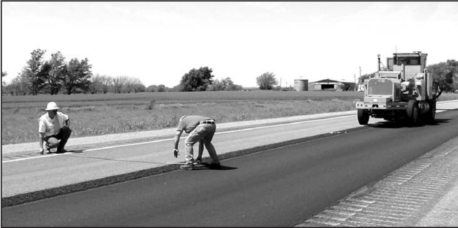
Centerline rumble strip construction on US-50 between Hutchinson and Newton.
