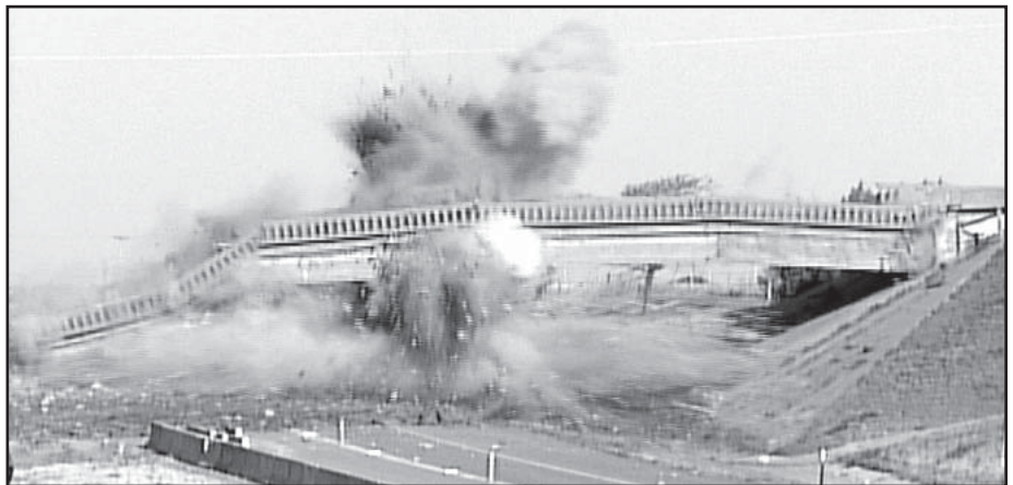
A Russell County bridge over I-70 near mile marker 179 comes crashing down on April 28 as part of a project to improve the interstate. One corner of the bridge had dropped more than six feet.
