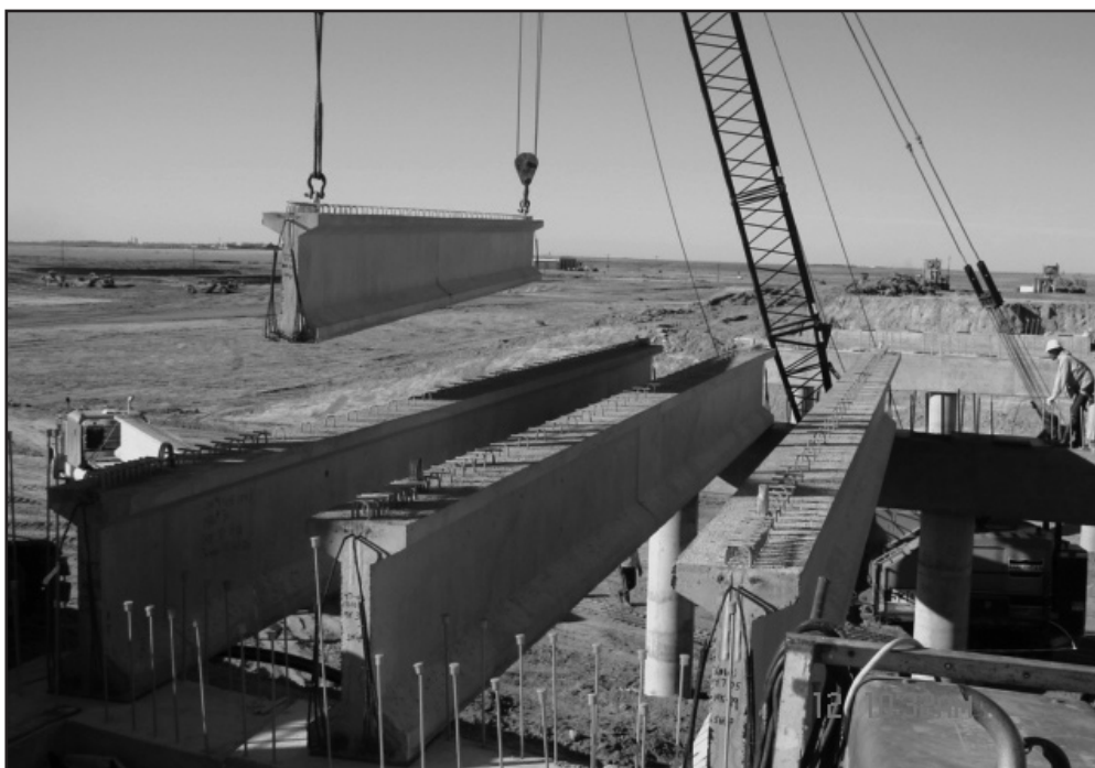
US-54 expansion work south of Liberal. Photo by Eric Jones
