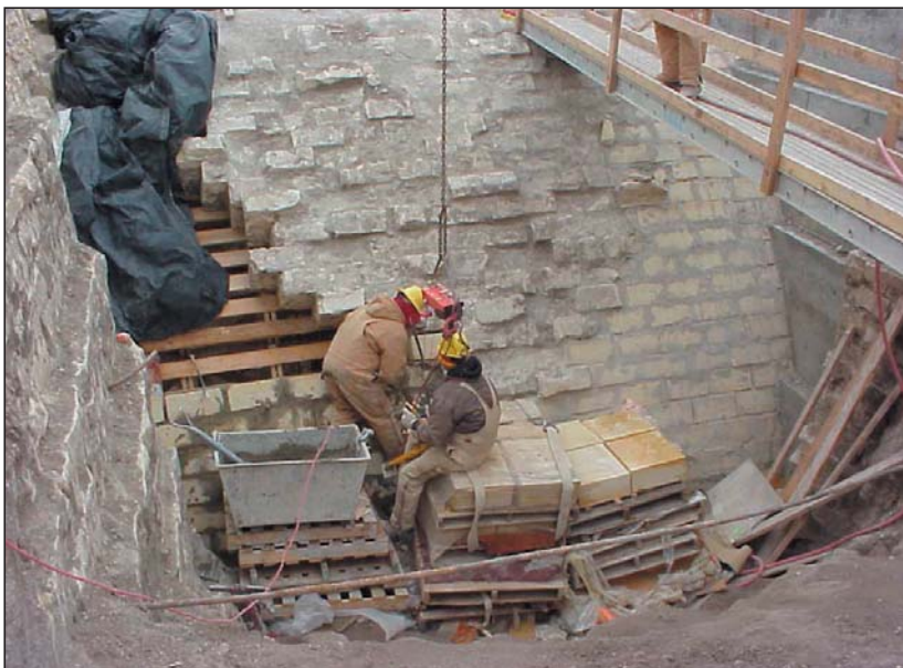
Workers replace some of the stones on the bridge.
