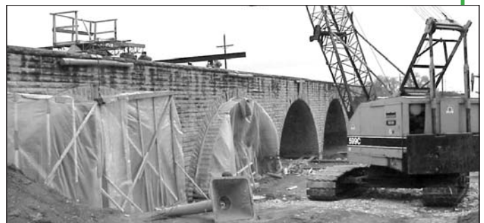
Renovation of the Fort Fletcher Stone Arch Bridge is nearing completion.
