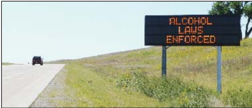
By early 2009, 15 Dynamic Message Signs will help inform motorists of road conditions and road closings along I-70.
