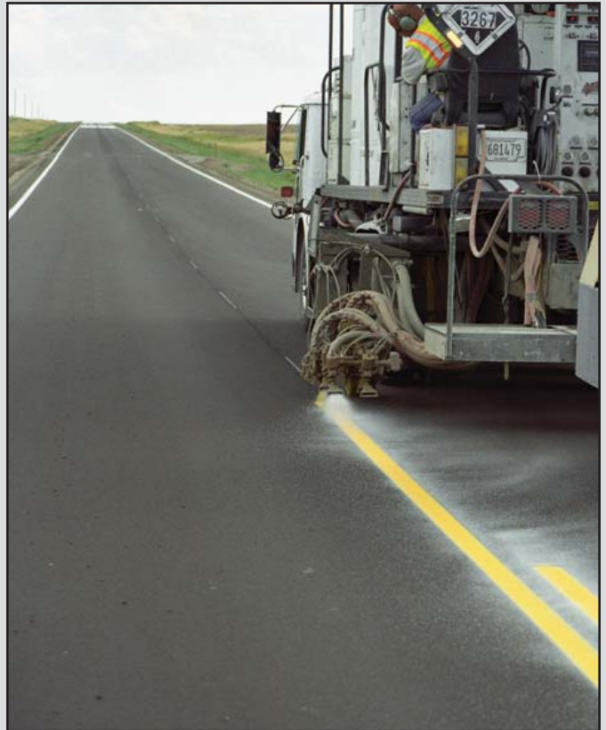
Center lines are placed on the new 16-mile stretch of K-23 pavement in Gove County. Photo by Kurt Weaverling
