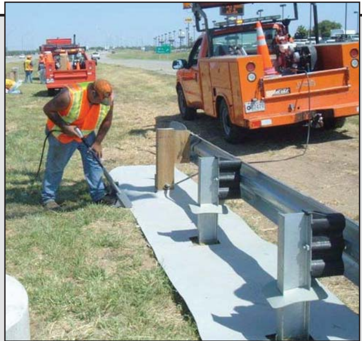
Equipment Operator Chris Riggs installs a roadside weed barrier along I-135 in Wichita.
