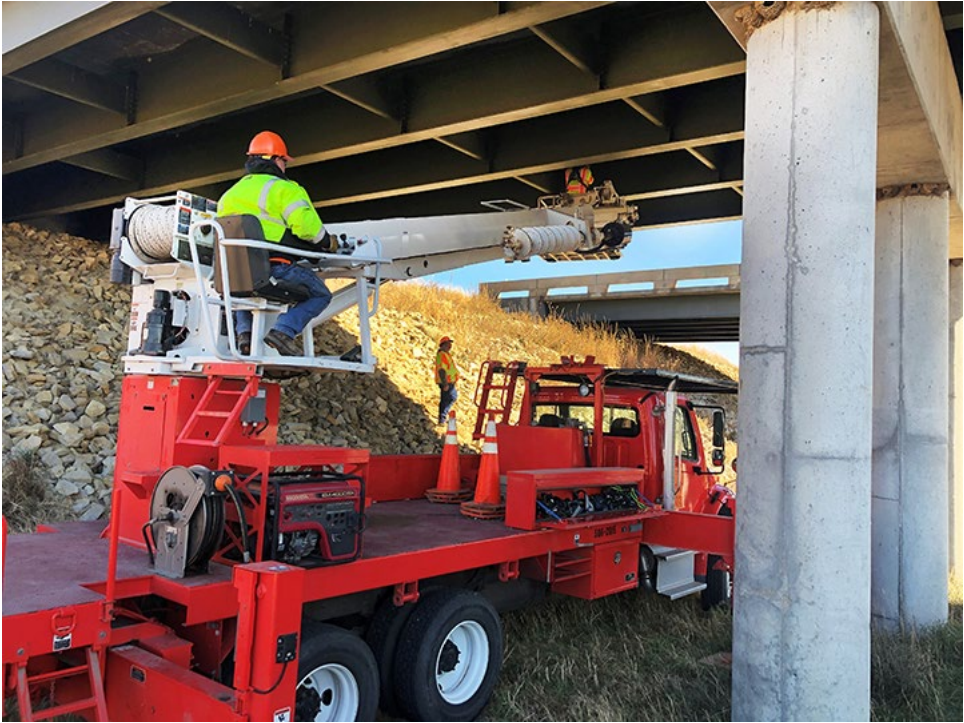
Left photo: Shannon Clarkson, Equipment Operator Senior on the District Specials Crew, operates the cherry-picker truck for Donnie Burkholder, Equipment Operator Specialist on the District Specials Crew. Burkholder is running wiring through the bridge deck for the new bridge sensor. Jeff Bogart, Equipment Operator Senior in Concordia, provides assistance from below. Right photo: Steve Schmidt, Highway Maintenance Supervisor of the District Specials crew, cuts out and removes the core of the failed bridge sensor. Photos by Ashley Perez, District Two
