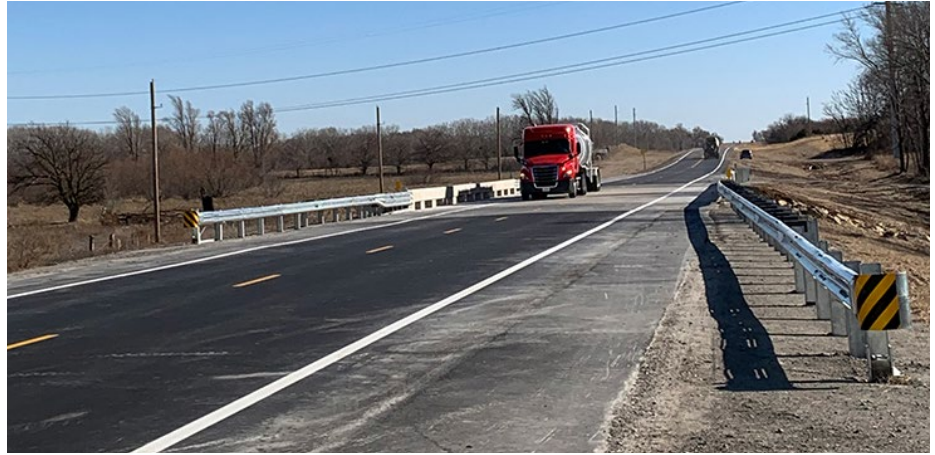
The new bridge on K-14 at Hunter Creek, near Kingman, is wider and offers better drainage. Photo by Jeremy King, District Five
