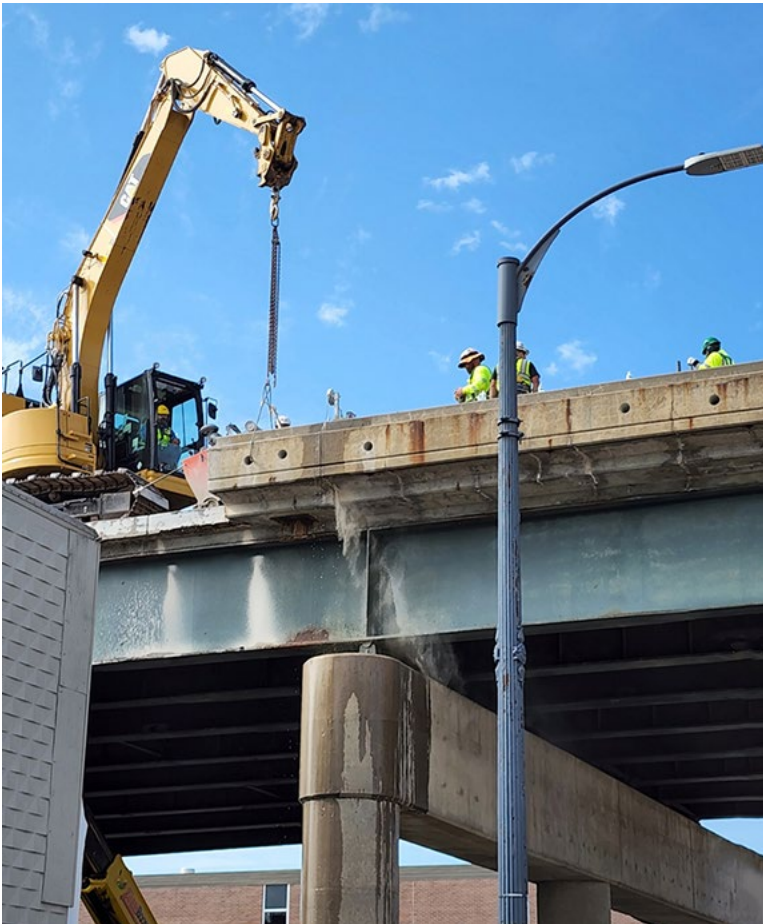
The photos above show different angles of the area along the Polk-Quincy Viaduct in Topeka where the concrete railing is being removed and replaced as a precaution after a section of concrete railing nearby had fallen in June. Photos by Kate Craft, District One, and KDOT Multimedia Services
