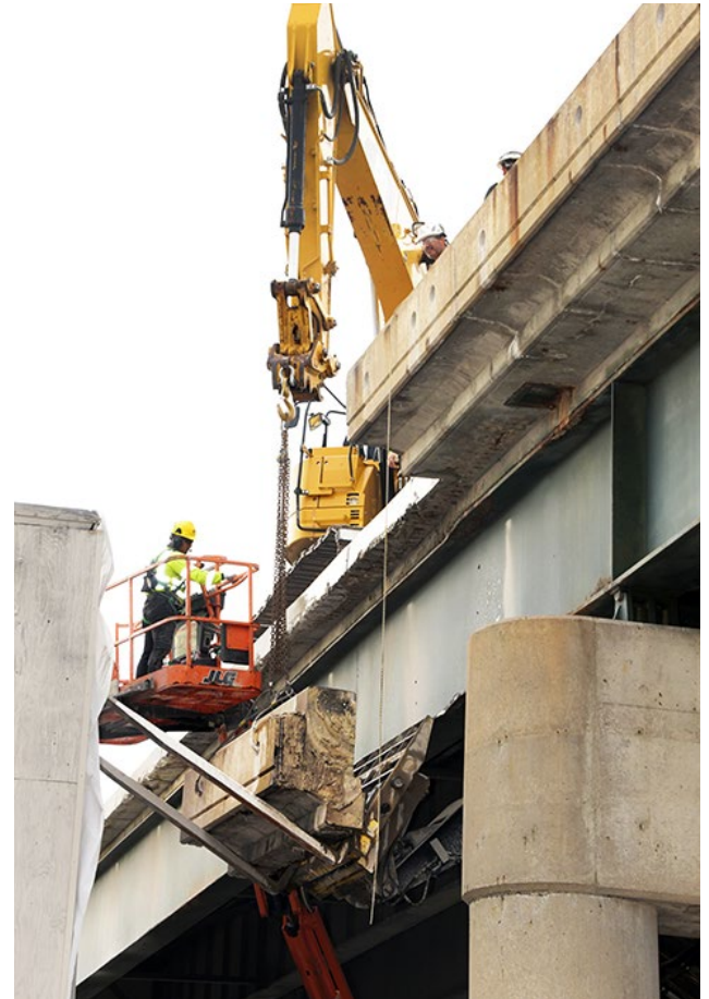
The photos above show different angles of the area along the Polk-Quincy Viaduct in Topeka where the concrete railing is being removed and replaced as a precaution after a section of concrete railing nearby had fallen in June. Photos by Kate Craft, District One, and KDOT Multimedia Services
