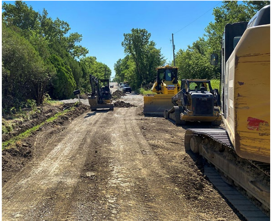
Grading is underway on West Maple Street at Independence. The roadway will be widened to 24 feet, and ditches will be moved away from edges of the street. Photo by Priscilla Petersen, District Four
