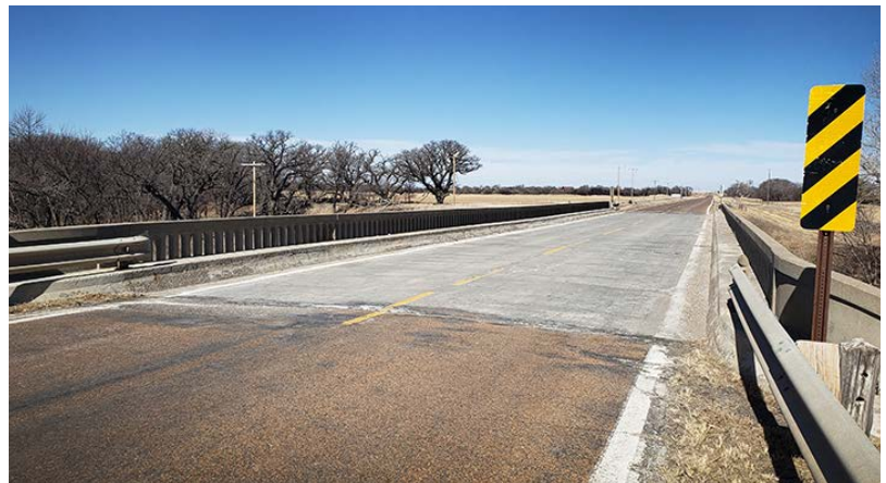
KDOT will replace the current continuous span structure, seen above and below, with a three-span, haunched slab bridge. Photos by Lisa Mussman
