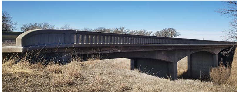
KDOT will replace the current continuous span structure, seen above and below, with a three-span, haunched slab bridge. Photos by Lisa Mussman
