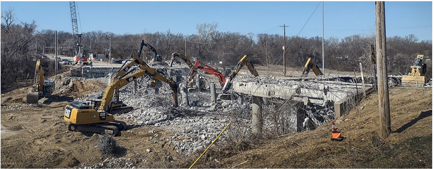
Crews demolish the existing bridge above the protected I-635 roadway. Photo courtesy of Clarkson Construction.
