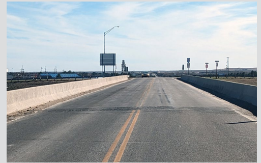
Reconstruction of the U.S. 183 bypass/I-70 interchange near Hays is one of several significant projects taking place in District Three during the 2024 construction season. Photo by Ashley Pfannenstiel, Hays
