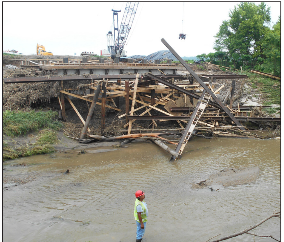
The photos above and below show the flash flooding damage that occurred in the past week in Nemaha County on the K-63 bridge work that was taking place as part of the bridge replacement project.
